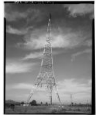
Chollas Heights Naval Radio Transmitting Facility, Tower 32, 6410 Zero Road, San Diego, San Diego County, CA Chollas Heights Navy Radio Station (Library of Congress image)
